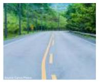
4. EDGE LINE – used to separate the outside edge of the road from the shoulder
