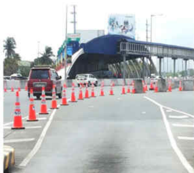
OBJECTS WITHIN THE ROADWAY
