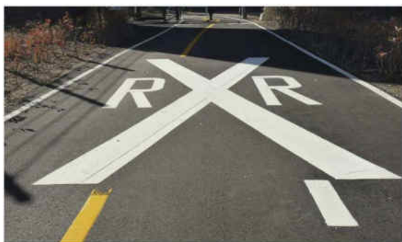
RAILROAD CROSSING AHEAD
